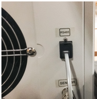
Figure D.12 - Chiller Communication Cable in RS-485 Port.
