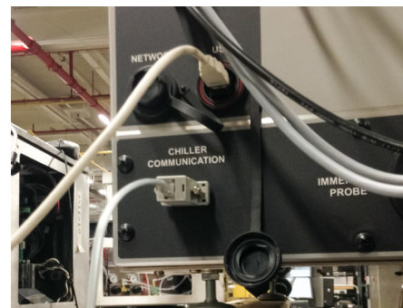
Figure D.13 - Chiller Communication Cable in BBR3 Chiller Communication Port.
