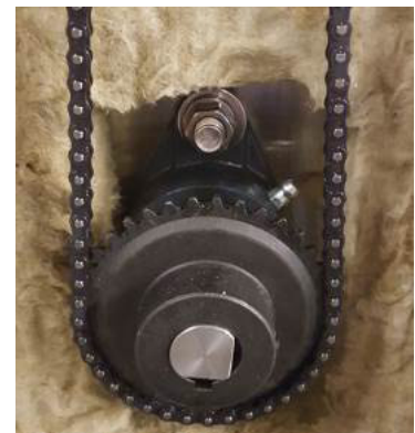
Figure H.3 - Exposed bearing at the bottom of the chain prior to greasing.
