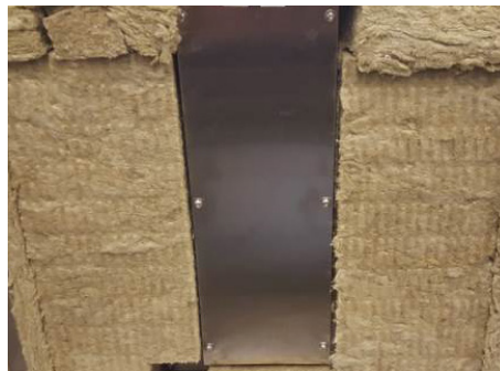
Figure H.2 - Remove the five screws on the rear cover.
