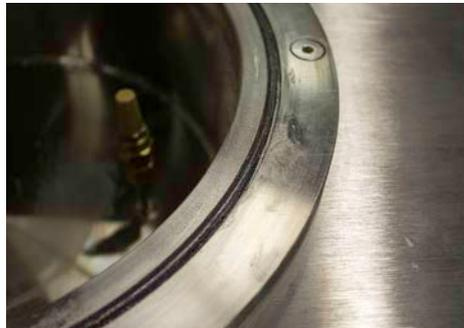
Figure D.1 - O-Ring in Place
