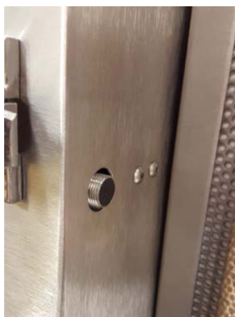
Figure G.3: RTFO door proximity switch
