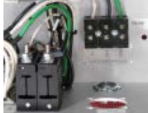
Figure C.2 - Interior Controller - Line Power Access Port
