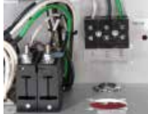
Figure C.2 - Interior Controller - Line Power Access Port
