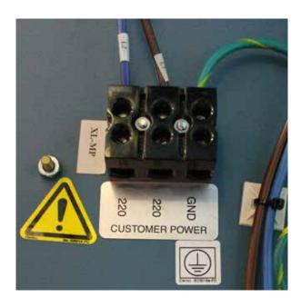
If the control cabinet is not supplied with a power cord, supply the incoming power to the terminal block.
